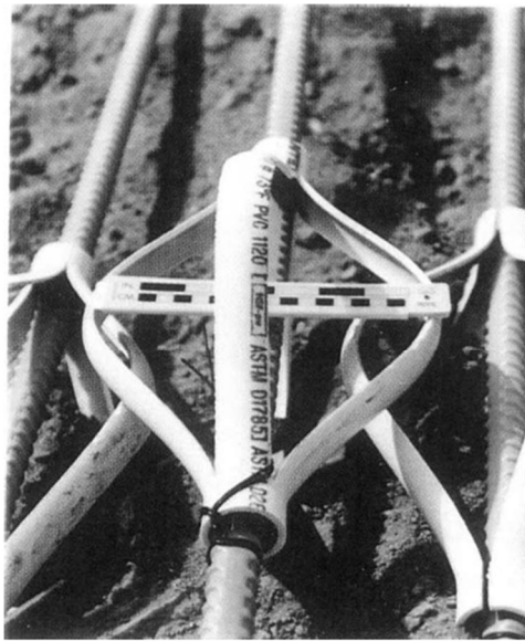
Figure 4.3: Typical PVC Centralizers Attached to a Nail Bar Prior to Nail Installation.
