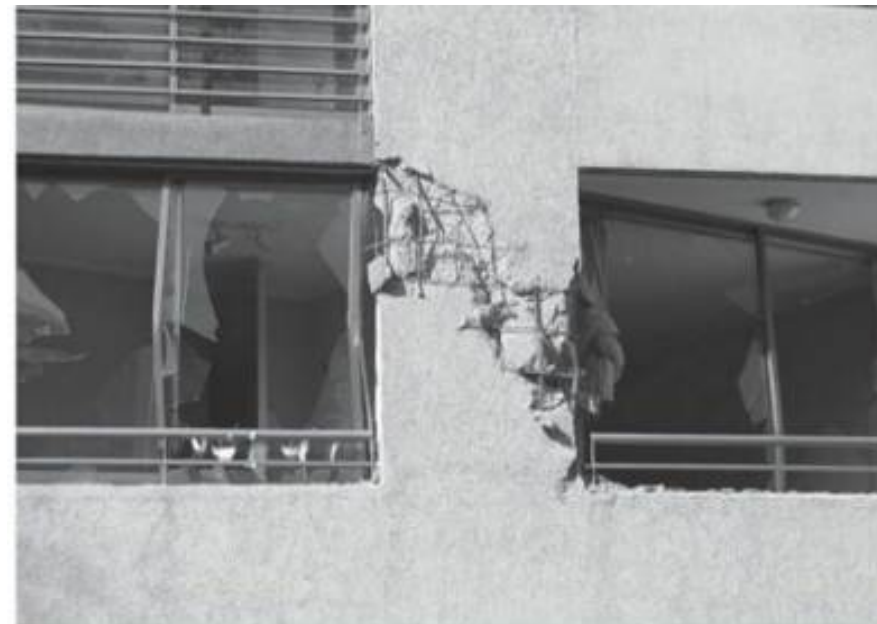
(b) Shear damage and onset of axial failure in vertical wall segment, 2010 Chile earthquake.
